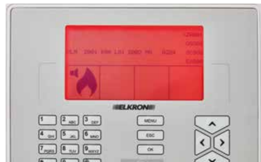
RED System in alarm
